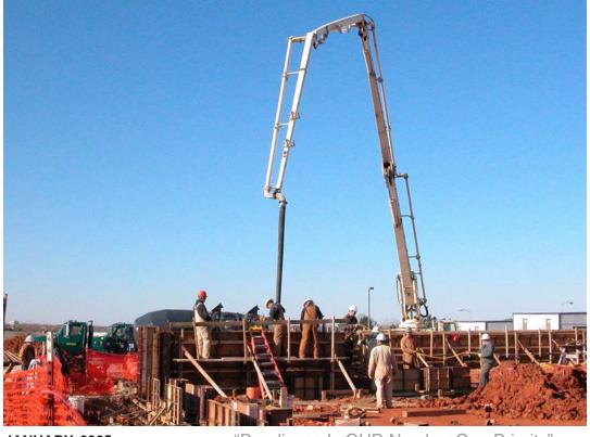
A large pumper truck is used to place the final grade beam concrete for the expansion of the 507th Civil Engineer **Building. Approximately** 150 cubic yards of concrete were used in the construction of the grade beam foundation system. The next step will be the concrete floor slab. Completion date for the entire project is scheduled for Spring 2005.
